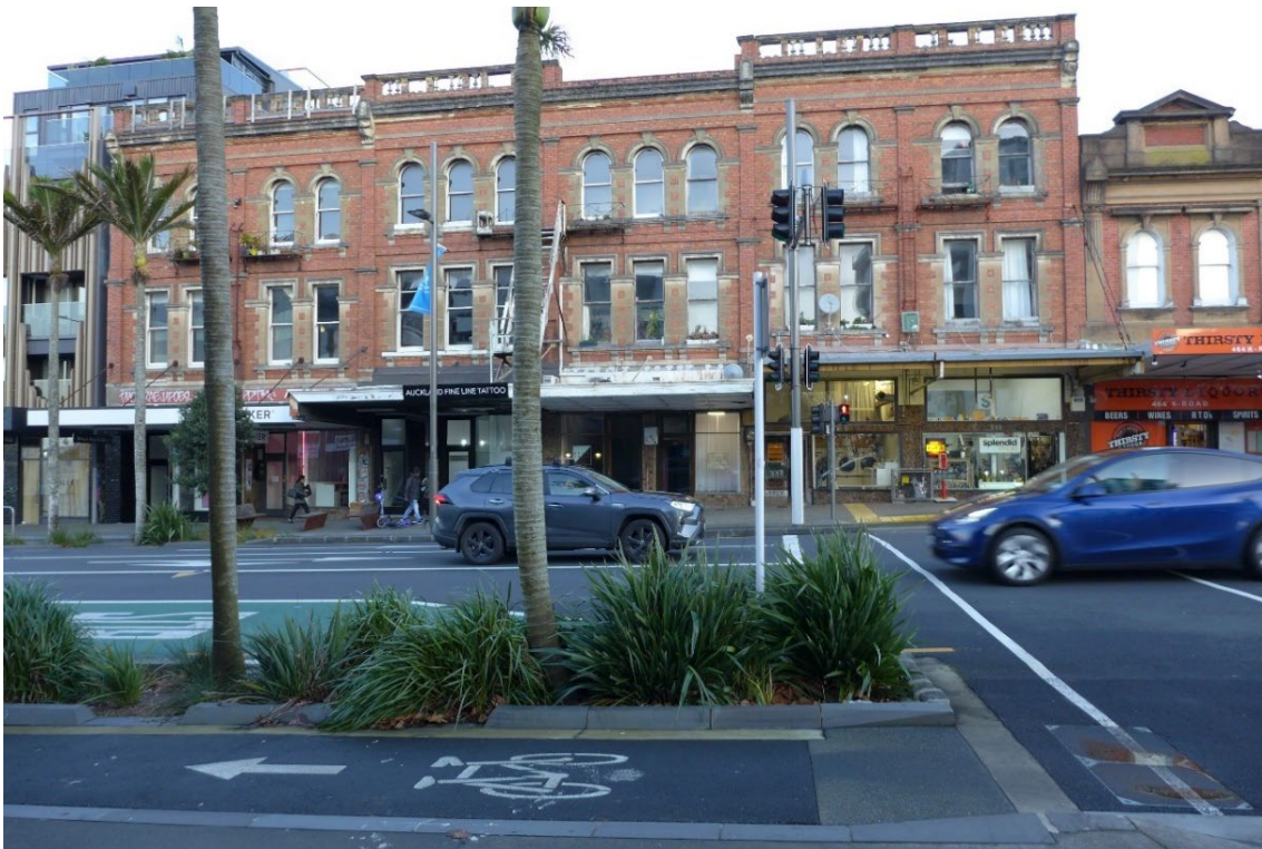
Figure 3 444-456 Karangahape Road. Although one balustrade is missing, the escalating cornice line is evident where the street level rises toward the west.
