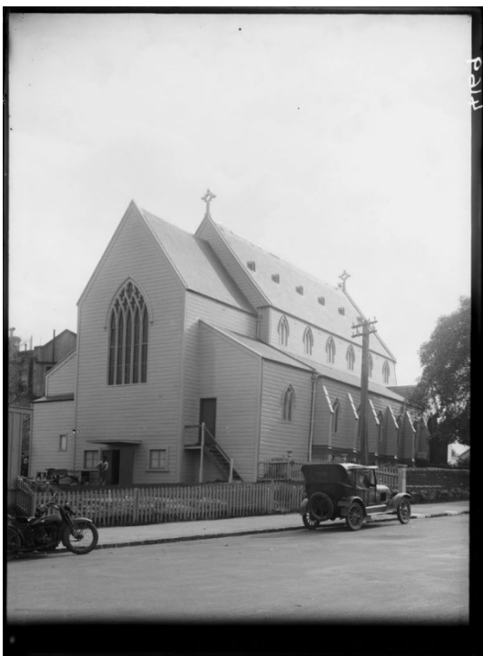
Figure 20: Rear view of Church of the Epiphany from Gundry St.
