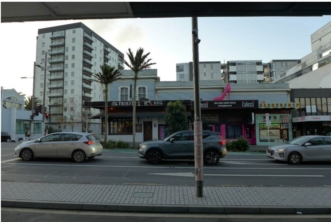
Figure 4 469 Karangahape Road (the Thirsty Dog) and neighbouring buildings. Single-storey buildings with high parapets match the scale of a two-storeyed building. Note the significantly taller built form behind the principal streetscape where the ground contours slope away sharply.
